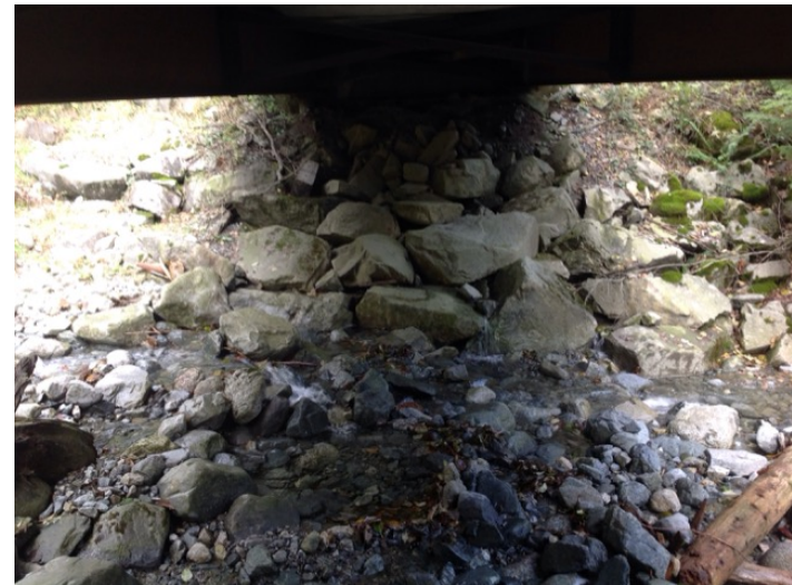
Left Bank Abutment when facing downstream
