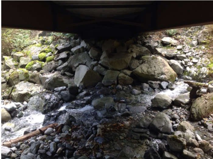
Right Bank Abutment when facing downstream
